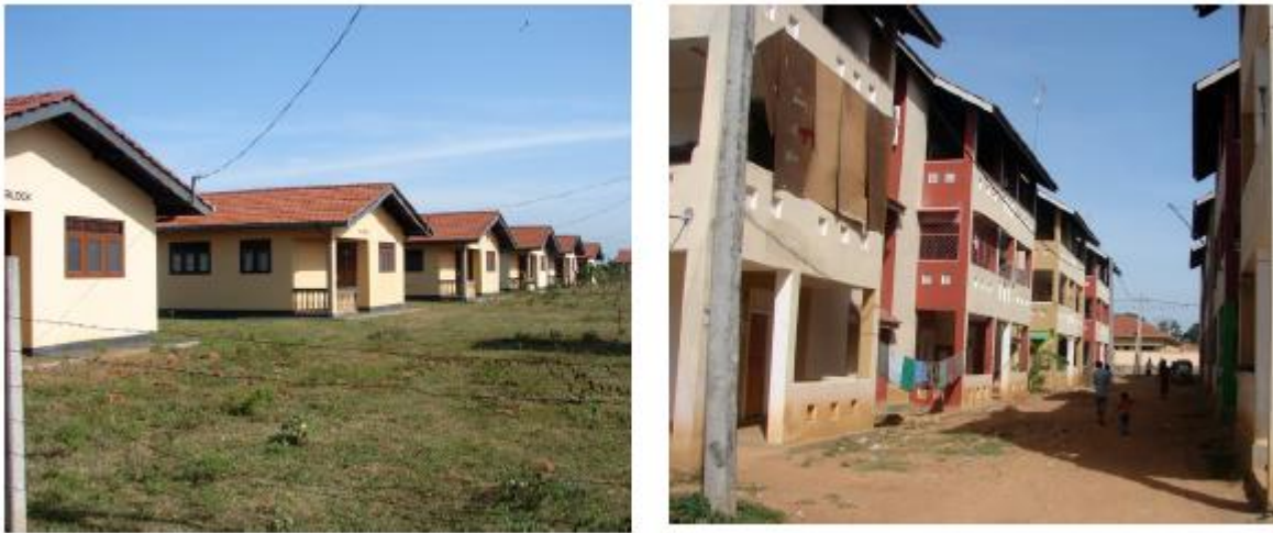
Figure 3&4: Contractor-built houses in relocated sites in Hambantota District, Sri Lanka (Duyne Barenstein, 2008)
