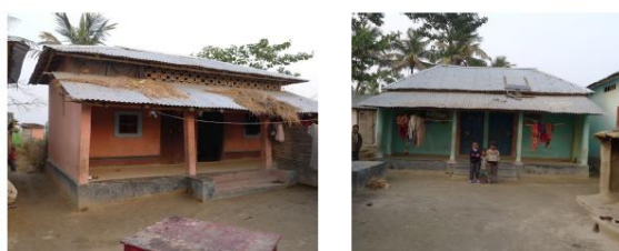
Fig. 23&24: Owner-built houses in Bihar, India (Duyne Barenstein, 2011)
