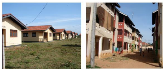
Figure 3&4. □ □ Contractor-built houses in relocated sites in Hambantota District, Sri Lanka (Duyne Barenstein, 2008)
